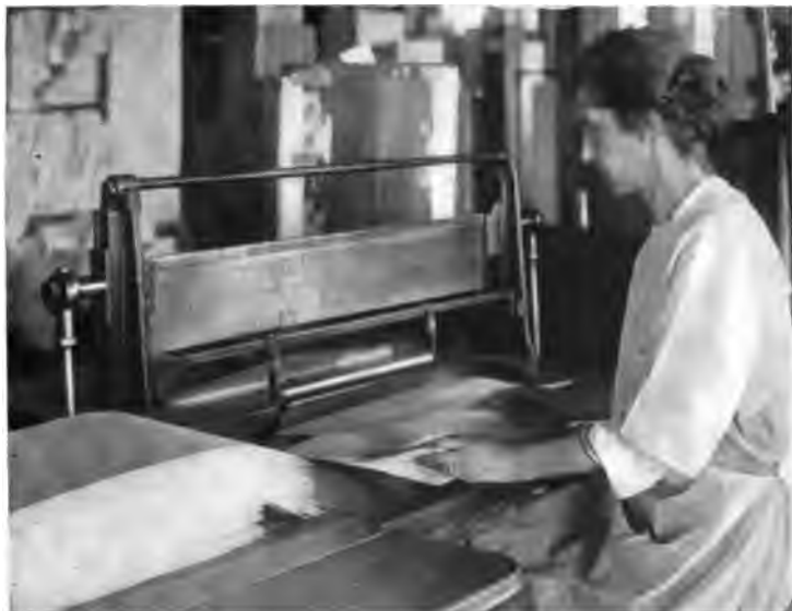
Fig. 1. Finger Guard (indicated by arrow) for Paper Folder.*
